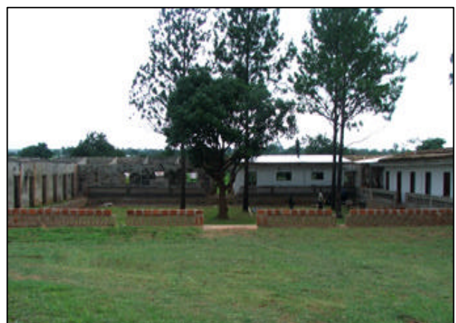
Here is a nice view of half the buildings. On the right are the volunteer/guest rooms. Directly in front are the two rooms for babies and toddlers and the reception/office room. On the left we plan to have an infirmary and a reading room with a good library as well as other rooms as the need becomes clear.
