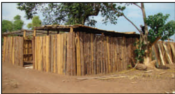
A chicken run being built with off-cuts
