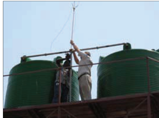
Here is Tom installing the first of 4 lightning rods for our property. Let the rains come.—We're ready!
